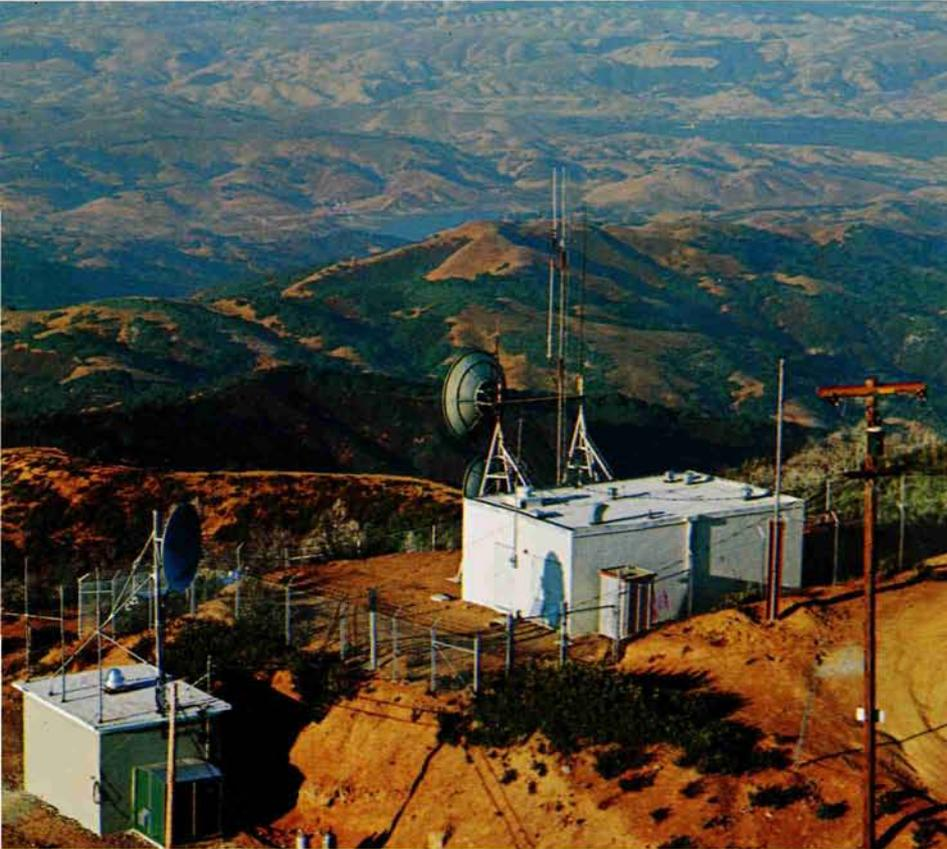
*Virtually all San Jose municipal departments depend upon two-way radio to do their jobs effectively. In order to make sure that radio coverage blankets every block of the city, San Jose communications experts have installed base station and microwave radio equipment and antennas on this mountain overlooking the valley.*
