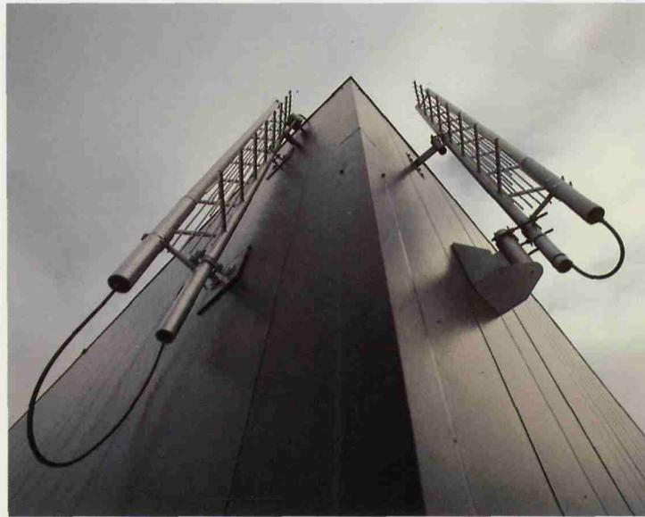
*These antennas are used in Motorola's Dyna T'A'C® experimental cellular system, which supports the use of Dyna T'A'C® portable telephones.*
